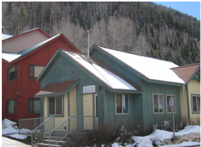
Daycare Center at Shandoka
